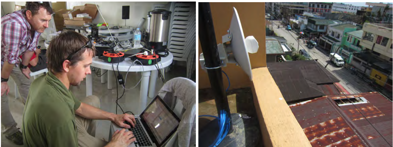
Left: Inveneo CTO Andris Bjornson configures wireless networking equipment in Tacloban. Right: Wireless Networking equipment on the roof of an NGO office in Tacloban.
